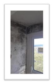
NW porch adjacent to dining room requires internal plaster to be removed and re-done. Due to previous water damage. (Use dust masks-mold)
